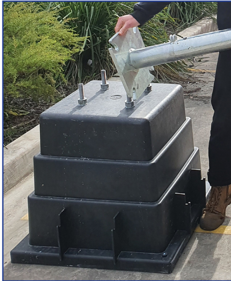
Fig. 2.3a Mounting pole onto concrete base
