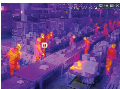
Fire Detection & Alarm Output
